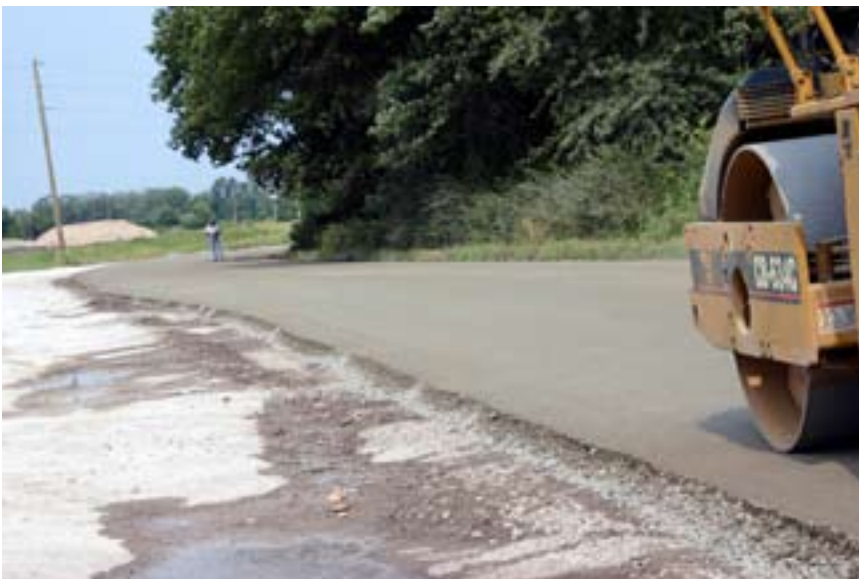
Above: RCC is placed by an asphalt spreader.
