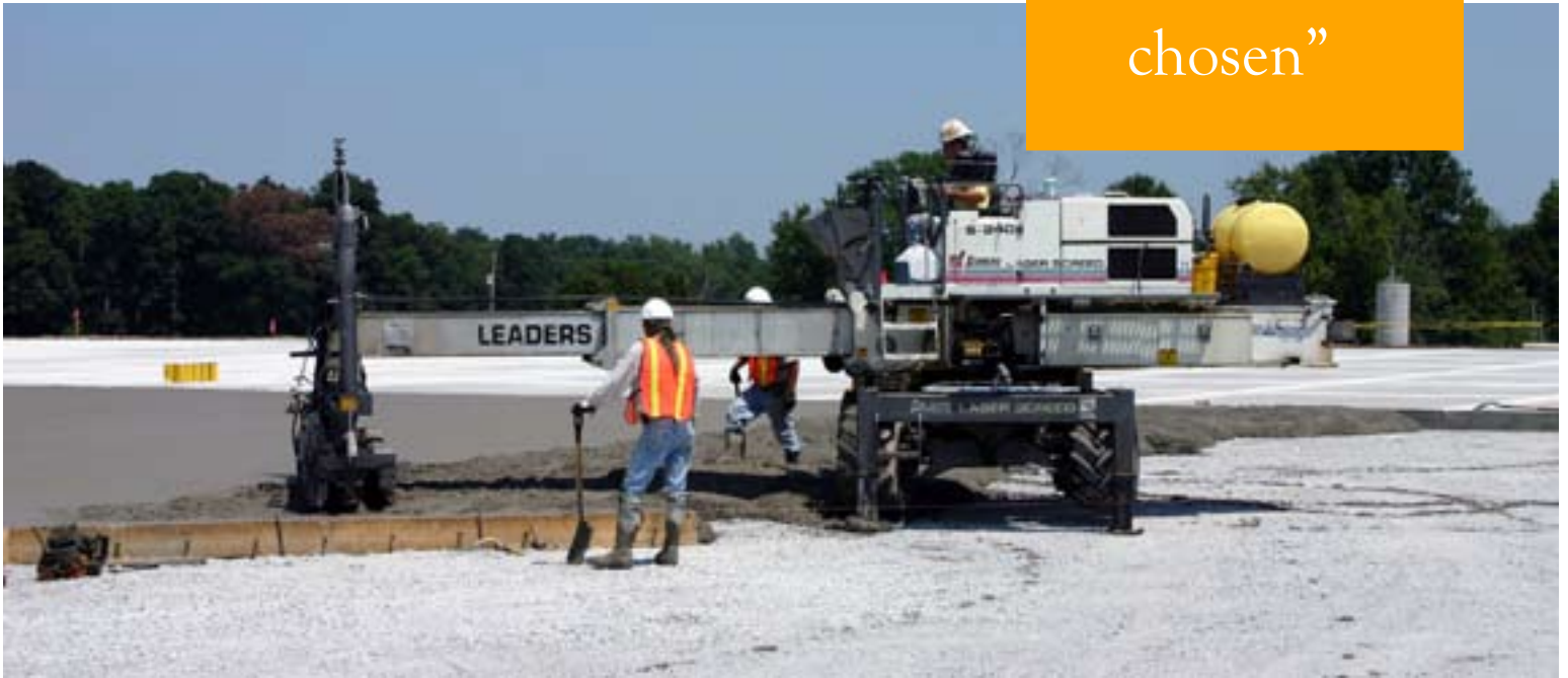
Top to bottom: Concrete is tested at the Wal-Mart jobsite; Concrete is being placed with a laser screed; A Prairie Farms truck parking lot was converted to concrete after a promotion effort by Doll's, Inc.
