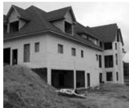
The Davis home, as seen from the backyard, provides a view of the two-story five car garage in this 9000 square foot concrete home. Forms were assembled and concrete was poured using the homeowner's crew.
