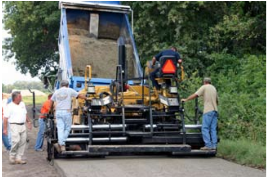
Above: RCC is placed by an asphalt spreader.
