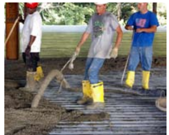
Workers are placing a floor mix that contains micro fibers.
