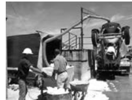
Proper dispersion of the fibers is essential in producing a mixture that is easy to finish and provides the needed structural characteristics. This blower does just that!
