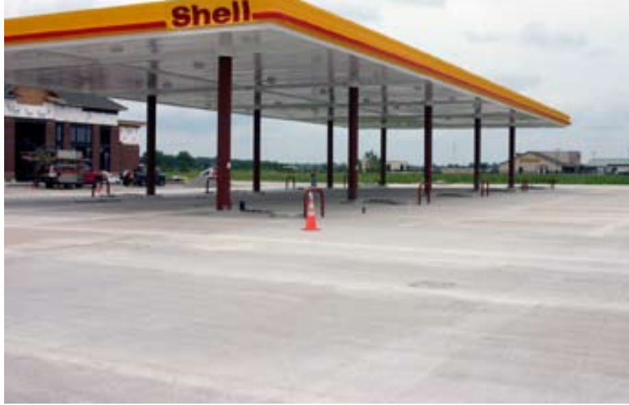
Shell station in Lincoln, Illinois, chooses concrete for entire project.
