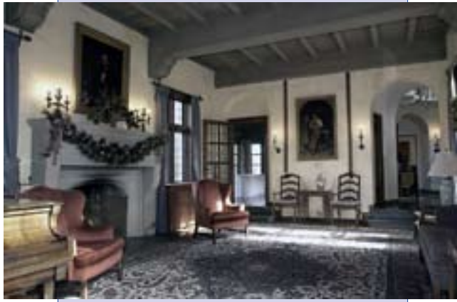
Concrete ceiling beams in the living room. Photo courtesy of ISU Marketing and Communications.
