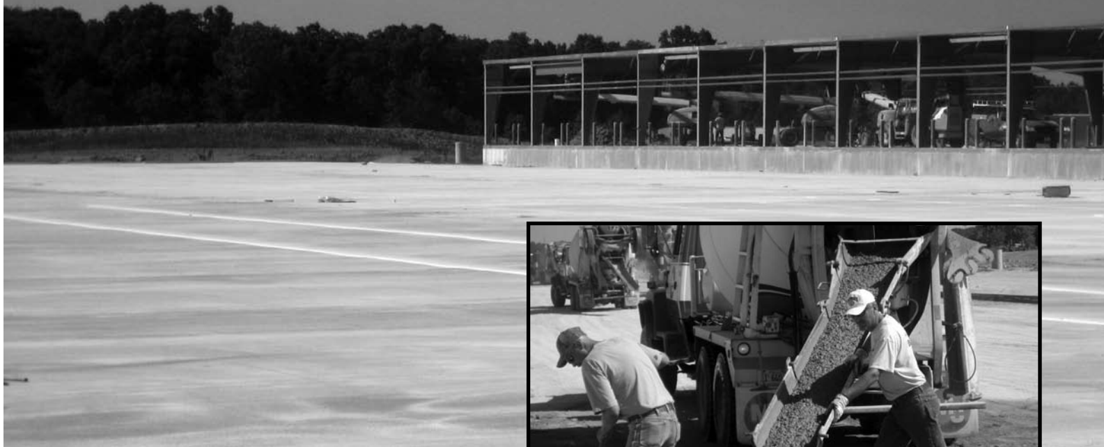
Above: Part of the completed pavement for FedEx in Effingham.
