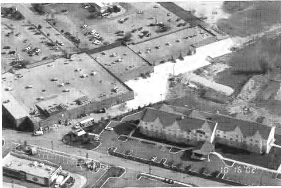
Above is an aerial view of the new pavement (the white area) behind Dominic's.
