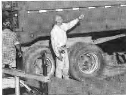
(Left) Len Swederski of Swederski Concrete supervises the concrete placement.
