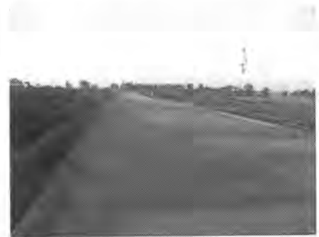
(Below) One of the concrete streets.
