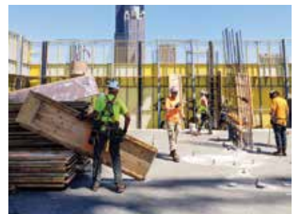
Forms are placed for construction of the 35th floor.
