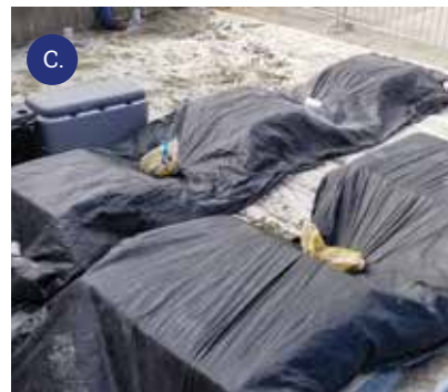
Figure 1: Casting and curing of slabs
