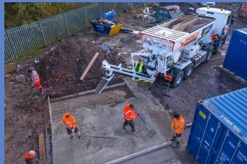
One of the biggest challenges facing Volumetric Mixer owners and operators is false setting concreting. The early stiffening of the mix can make it completely unworkable and
