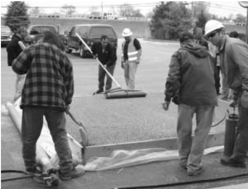
Above: IRMCA is now authorized to offer pervious technician certification. Here technician hopefuls practice on a test slab.
