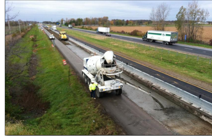
I-69 rebuild north of Indianapolis
