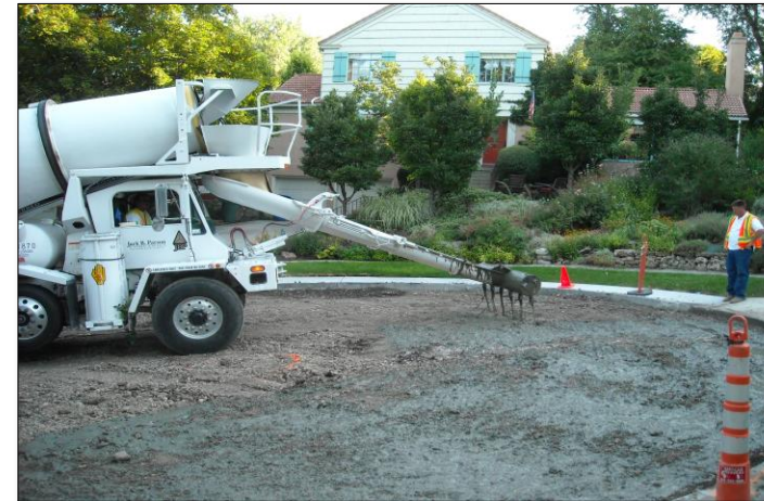
Slurry spreader attached to RMC truck
