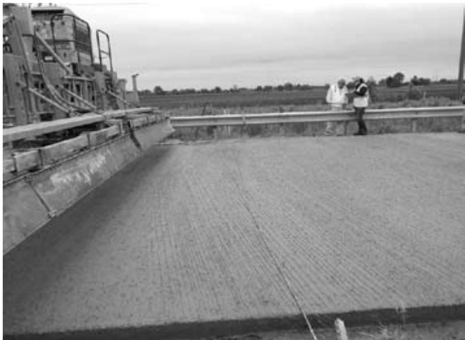
these were eased significantly by the lack of having to work around, over, and occasionally under the stringline. There were initial concerns about the ability to tine the surface given the incorporation of the fibers, but a test placement completed the prior week at D's yard proved the concerns largely unwarranted. There was no unusual difficulty finishing or tining the surface. Curing was applied immediately upon completion of the tining operations prior to jointing the pavement.
